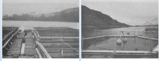
Fig. 25 Square timber-framed floating cages
